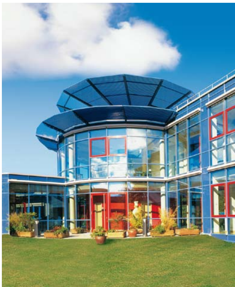
The Technology Centre in Ahrensburg, near Hamburg
