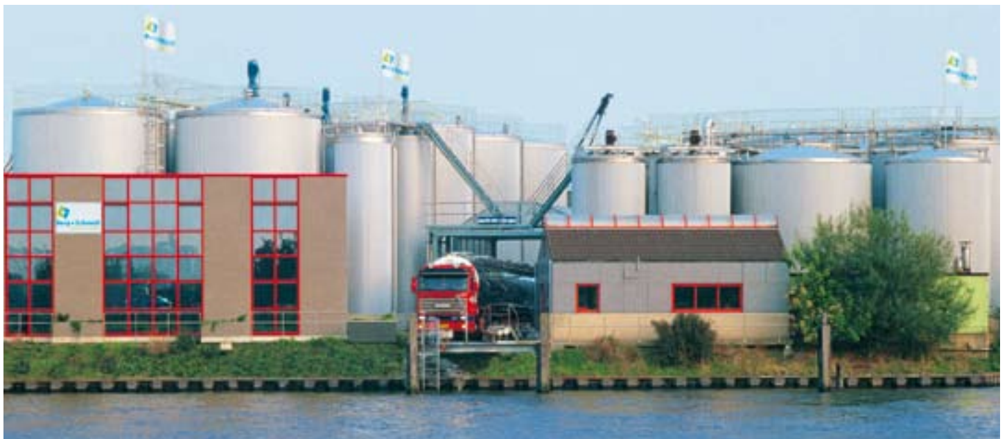
The stainless steel tank farm in Ouderkerk near Rotterdam, Netherlands
